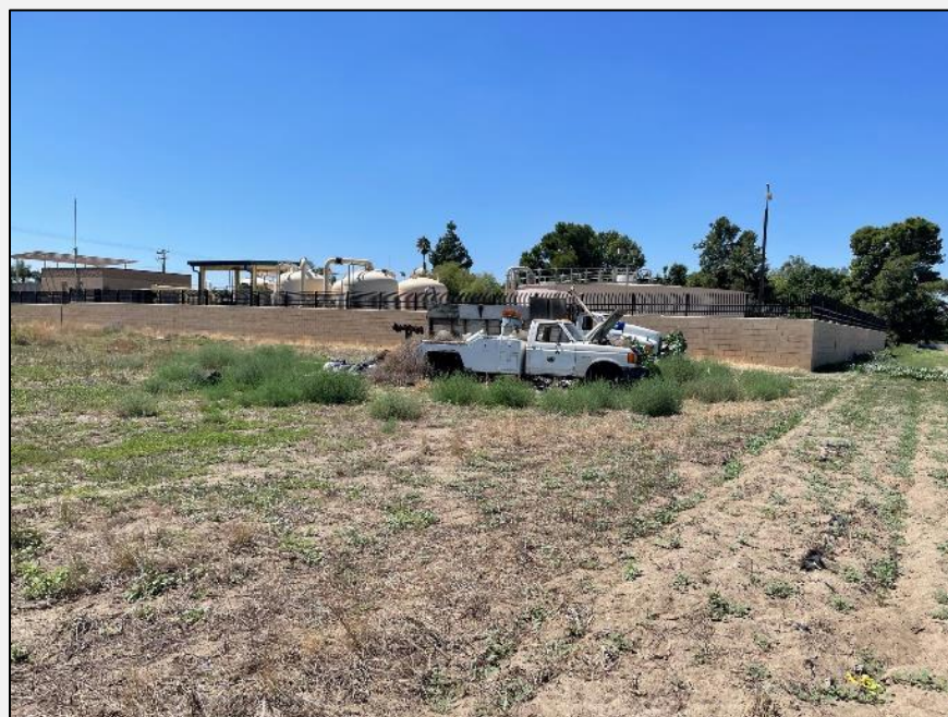
Exhibit 3. Overview of western portion of Treatment Plant APE; view to southwest.
